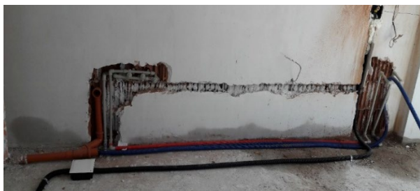
(b) Real done domestic gas installation – the corrugated pipe is black
