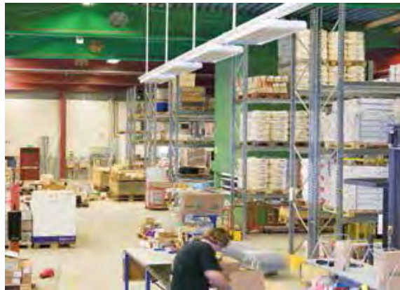
Fig. 4. Zone heating with radiant heater
