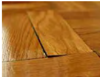
Fig. 3. Inflated flooring due to high inside humidity.
