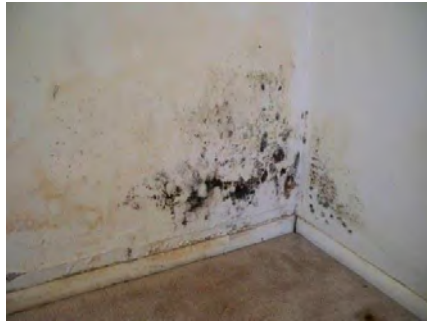
Fig. 1. Damaged wall by mold. Fig. 2. Corrosion on steel reinforcement.
