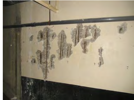
Fig. 1. Damaged wall by mold. Fig. 2. Corrosion on steel reinforcement.
