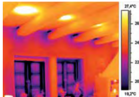
Fig. 6. Thermal bridges between the roof beams and adjacent walls.
