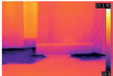
Fig. 7. Moisture intrusion in floor.
